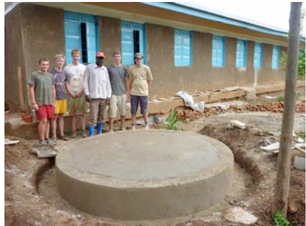
Base for new water storage tank built by Scouts.
