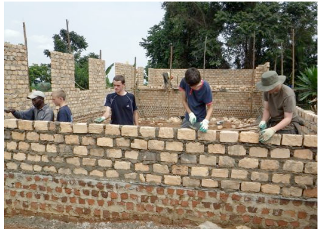
Scouts bricklaying with the help of local builders.
