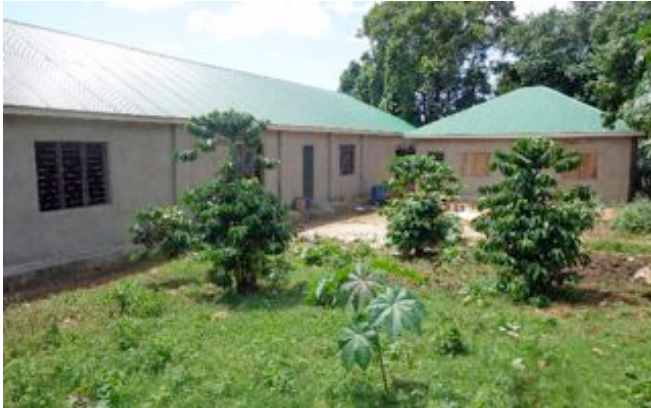
Buildings constructed by Berkshire Scouts alongside local builders. Classrooms (left) and kitchen/diner (right).
