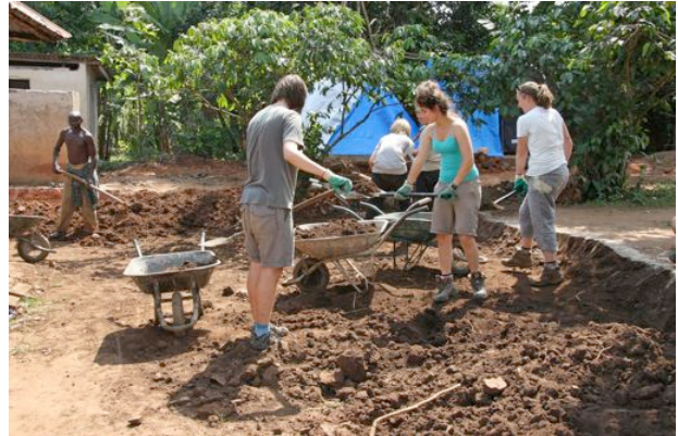
Scouts moving tons of soil by wheelbarrow!
