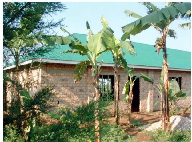
Photograph shows the roofing of the multi-purpose building (Bukeka) has been completed by local builders
